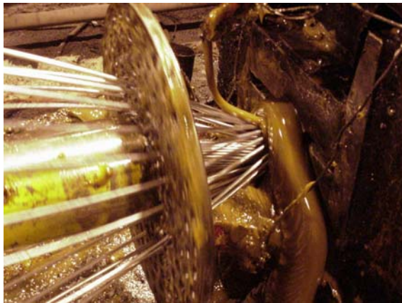
Figure 3. Application of preservative.
