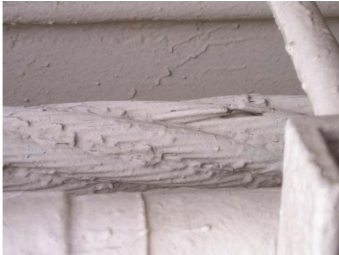
Figure 5. Fretting of suspender ropes.
